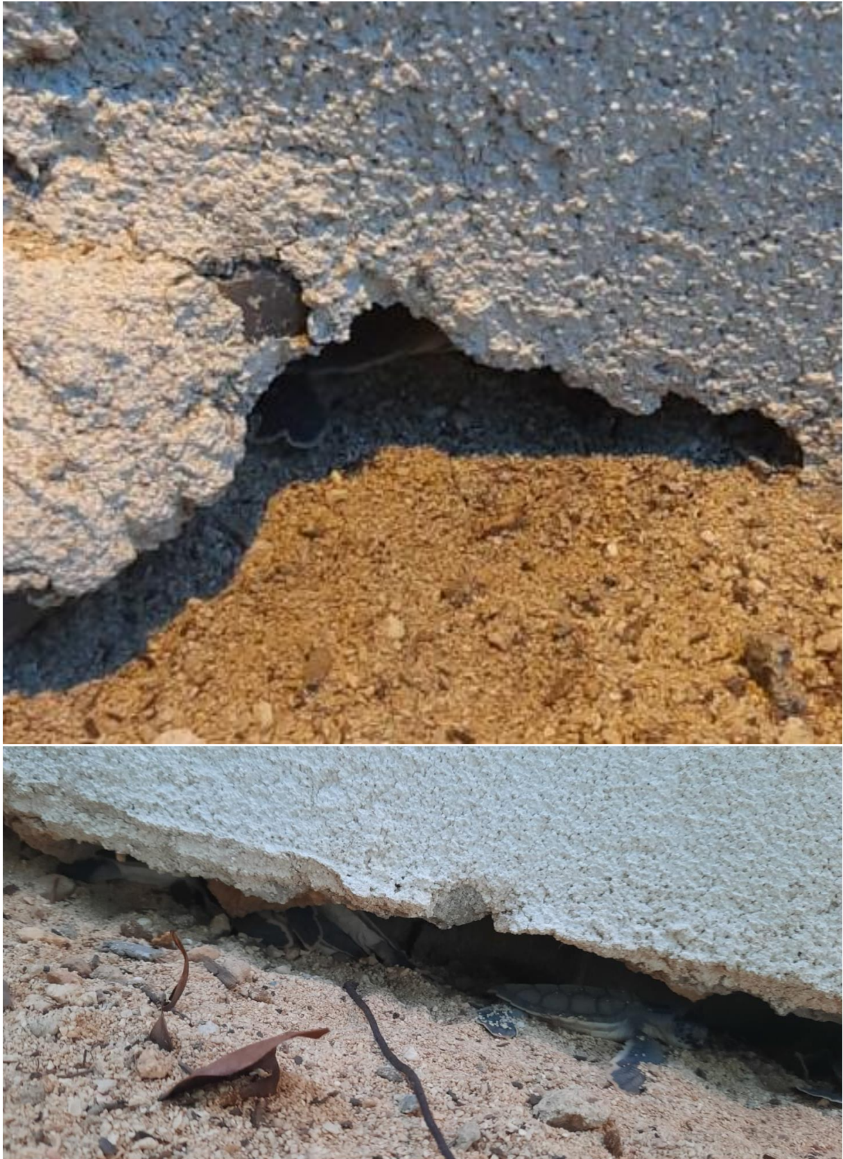
Figure CS1.3. Sea turtle hatchlings that became misoriented by artificial lighting and then became stuck within the seawall at the case study site 5 .
