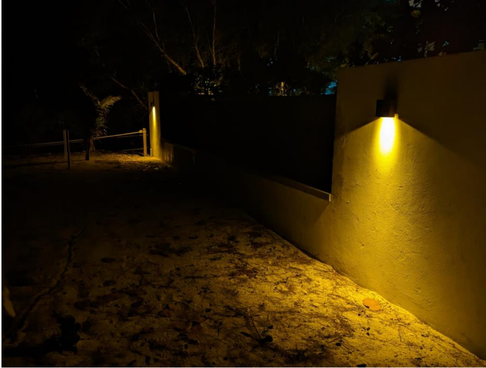
Figure CS1.1. Bright exterior lighting that directly illuminates the sand at the case study site 5 .
