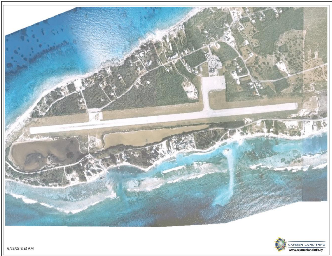
Figure 6. By 1994, the ponds have been heavily impacted by the airport construction (Source: Cayman Land Info, 1994).
