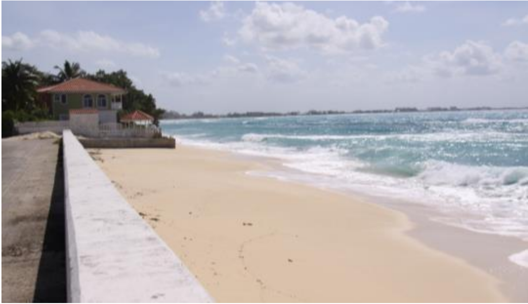
Picture 4: The site in November 2010 during a period of inclement weather. The seawall has only recently been constructed.
