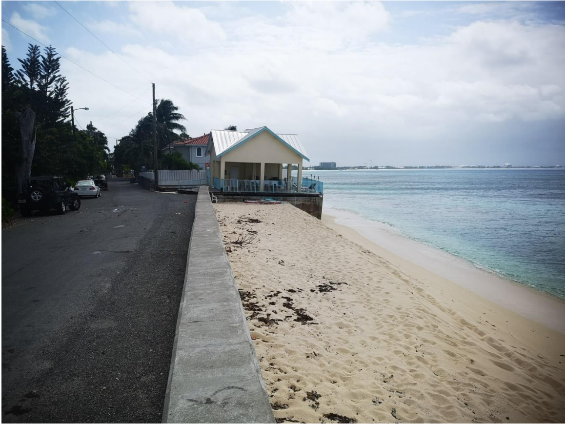
Figure 16: The site in March 2021, showing a steeper reduction in the volume of sand on the beach.
